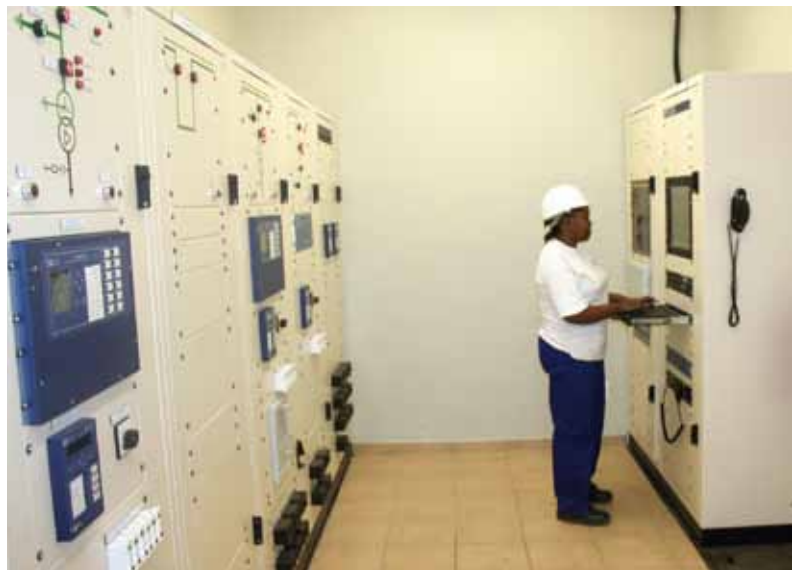
Photographs of a Remote Terminal Unit (RTU) Cabinet at Manzini North Substation
