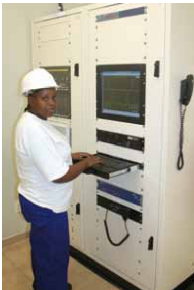
Photographs of a Remote Terminal Unit (RTU) Cabinet at Manzini North Substation
