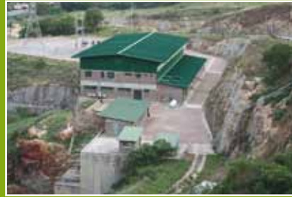
Maguga Power Station
