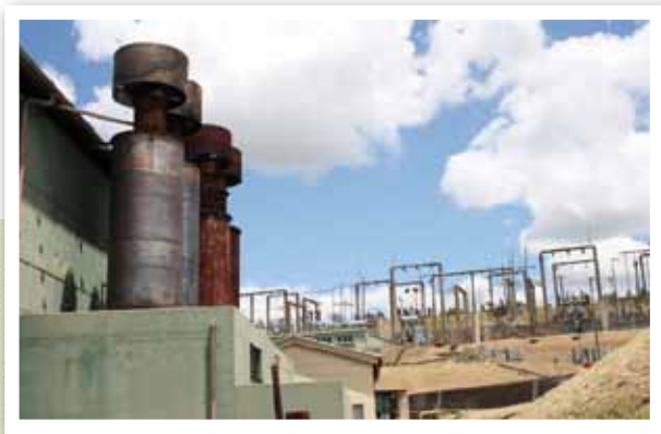
Background: Edwaleni Power Station under construction – 1963. Left: Edwaleni Power Station – 2011.
